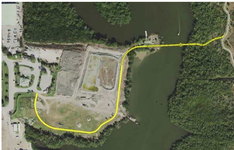
Boardwalk and Bridge alignment
